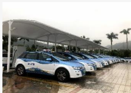
Taxi Charging Station
